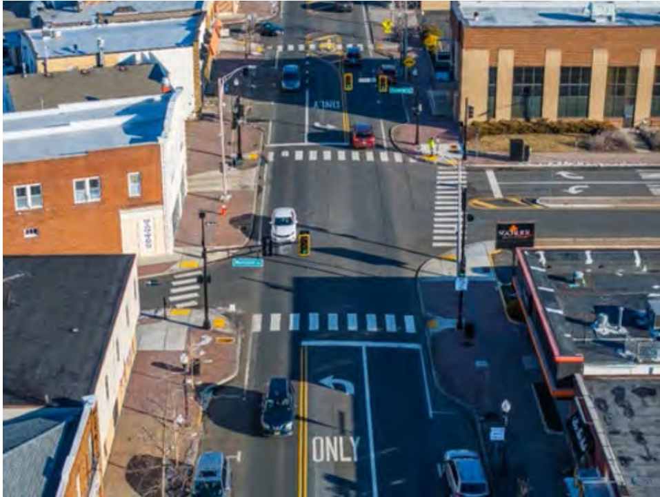
High Visibility Crosswalks / Detached Curb Extensions
