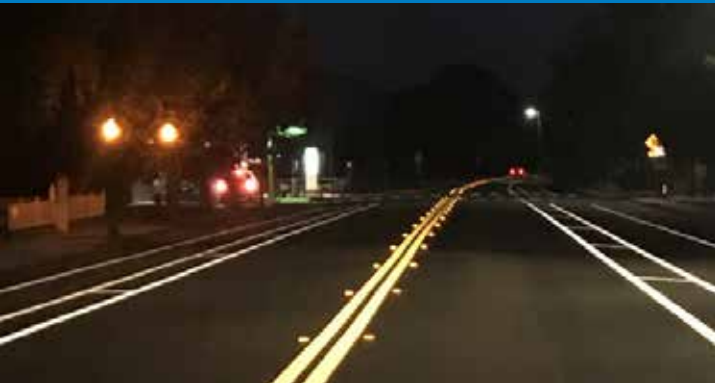
Raised Pavement Markers (RPMs)
