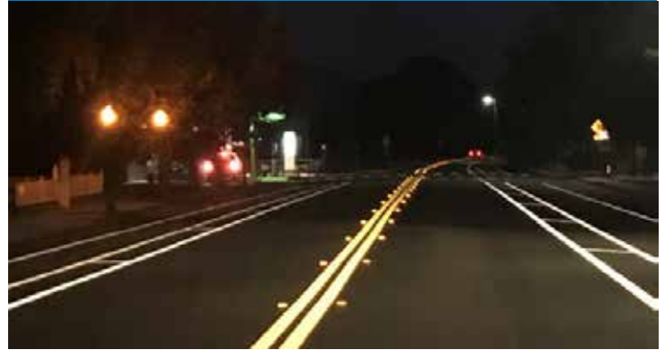
Raised Pavement Markers (RPMs)
