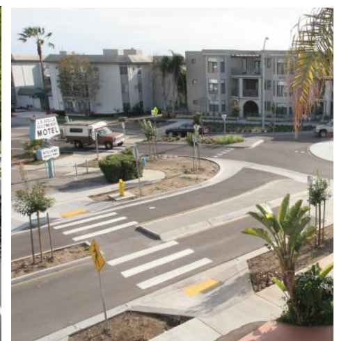
Median and pedestrian refuge island near a roundabout. Source: www.pedbikeimages.org / Dan Burden
