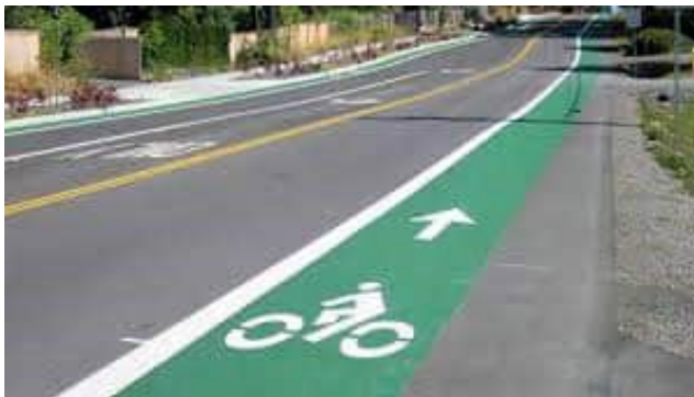
Unprotected – on shoulder
