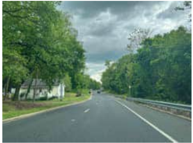
Between S. Pearl Street and Baltimore Avenue, Grove Street is two lanes southbound.
