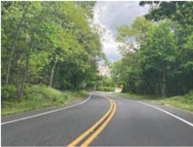
The culvert collapse on South Avenue has diverted traffic onto Grove Street, which was converted into a two-way street between Rocap's Run and Baltimore Avenue.
