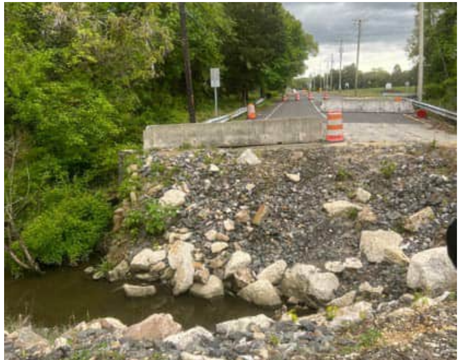
The culvert on South Avenue crossing Rocap's Run partially collapsed in 2020.
