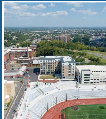
Hinchliffe Neighborhood Restoration Project (Paterson)
