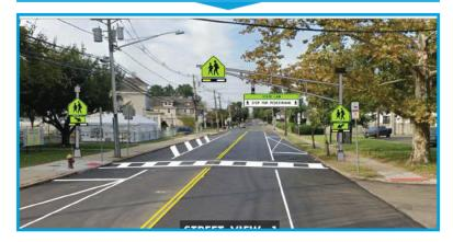
An RRFB is a proven safety countermeasure with a pedestrian crash reduction of up to 47%. A median pedestrian island is also a proven safety countermeasure with a pedestrian crash reduction of up to 46%.
