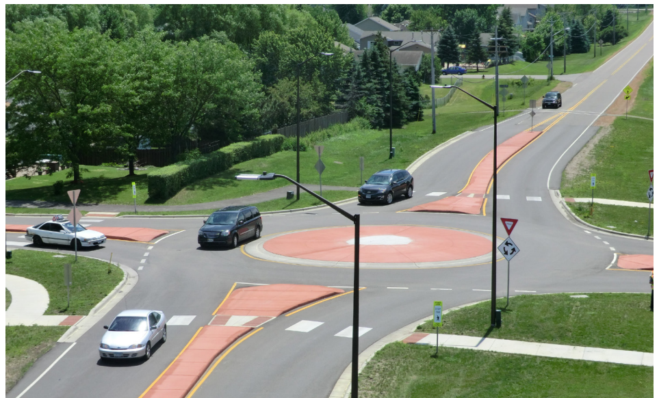
Example of a single-lane roundabout. Source: FHWA
