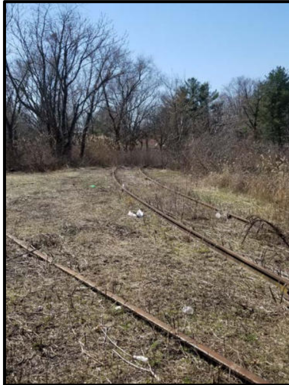
Figure 15 Salem Branch near Former Rail Yard
