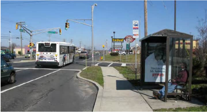
Access to the bus stop at Route 42 and Greentree Drive in Turnersville was improved with a bus pull out and sidewalks. Image: Parsons Brinckerhoff
