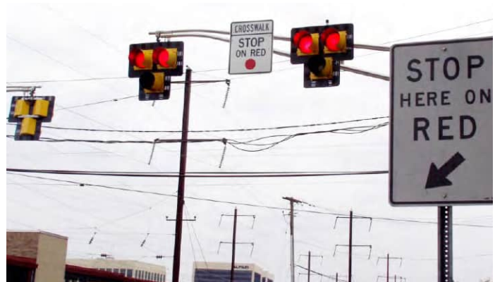
NJDOT installed a pedestrian hybrid beacon, or HAWK signal, at Route 27 in Woodbridge near the Metropark Rail Station. Image: NJDOT
