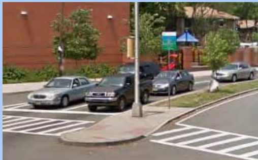
Pedestrian Refuge Area at the intersection of South Orange Avenue and Maybaum Avenue in Newark, NJ. Image: RBA
