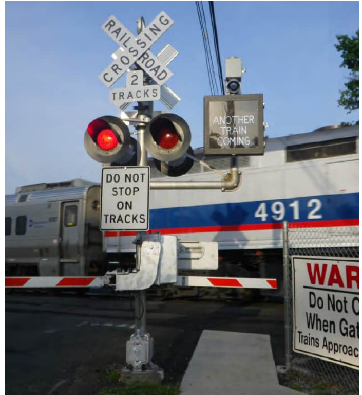
“Another Train Coming” pilot program at Plauderville Station in Garfield. Image: Marco DeSilva, Volpe Center
