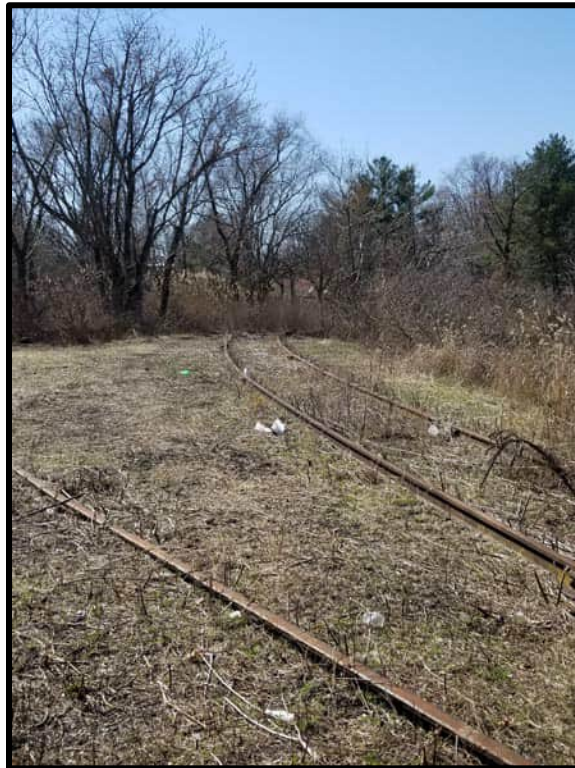
Figure 15 Salem Branch near Former Rail Yard
