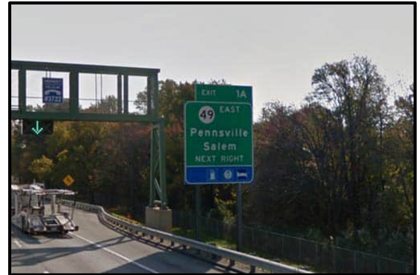
Figure 23 Current Sign for Eastbound Traffic on I-295
