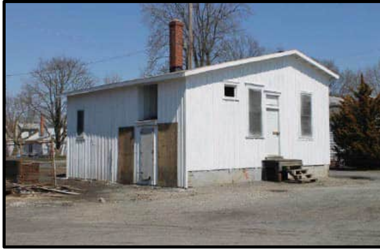
Source: Reconnaissance-Level Architectural Survey of the Salem Railroad, Salem County, 2014.
