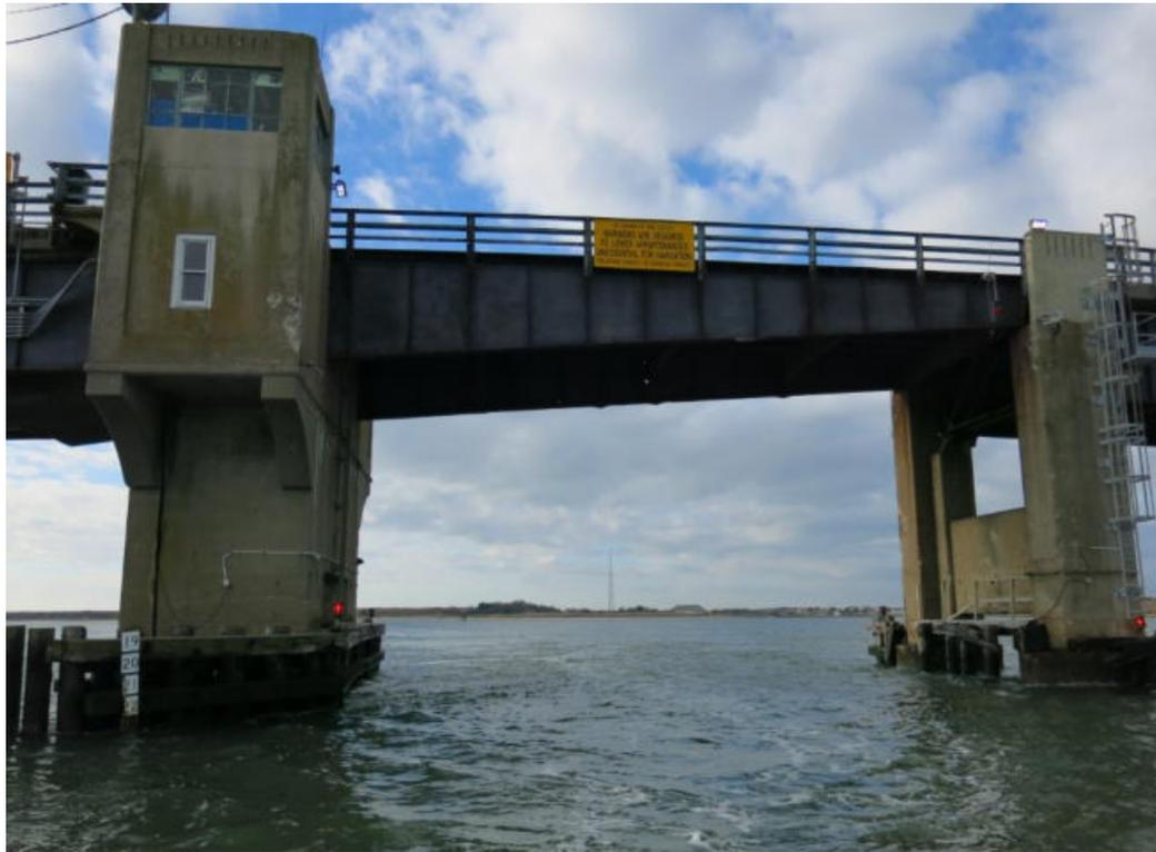
**Figure 22: Existing Bascule Span**
