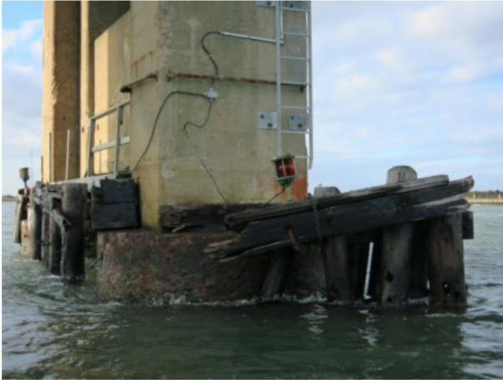
**Figure 12: Timber Fender**
