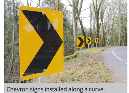
Chevron signs installed along a curve.
