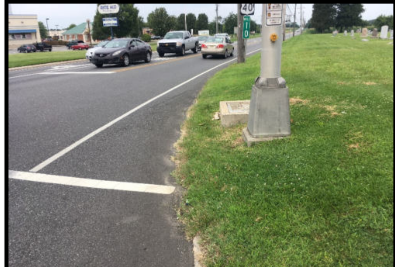
Looking west at the Eastbound Approach
