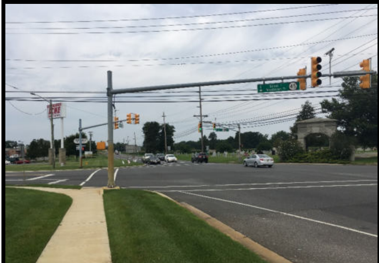
Looking west towards US Route 40
