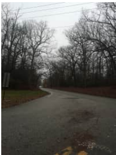
Photo 12: West Park Drive east of Mayor Aitken Drive
