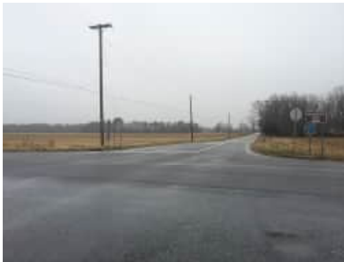
Photo 8: Northbound Approach of Hogbin Road
