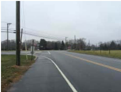
Photo 1: South Woodruff Road south of Rosenhayn Avenue, east intersection
