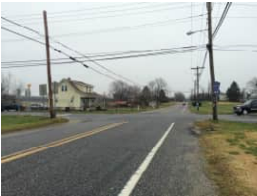
Photo 10: Morton Avenue north of Lebanon Road
