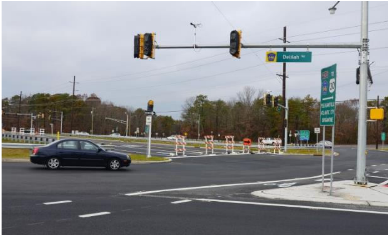
Photo 2: Looking northwest at newly constructed "Airport Circle", November, 2011 (McKelvey, 2011)
