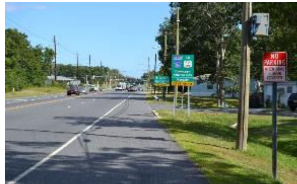
Photo 3: Looking EB on Delilah Road west of Airport Circle
