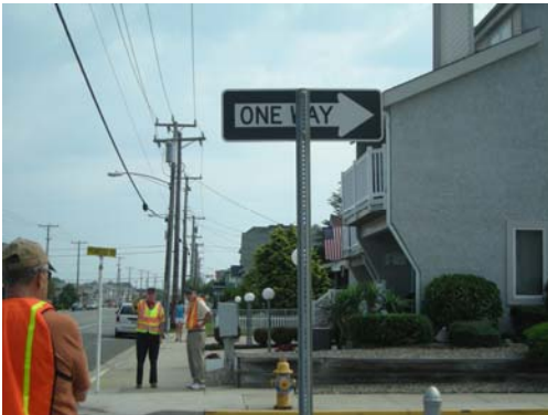
PICTURE 7: ONE (1) ONE-WAY SIGN MOUNTED INSTEAD OF BACK- TO-BACK MOUNT, NON- BREAKAWAY POST AT PRIMROSE AVENUE
